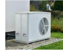
$$1 \text{ kWh} + 3 \text{ kWh} \\ = 4 \text{ kWh th}$$
